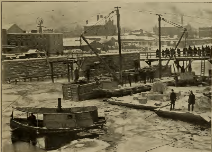
STATE STREET BRIDGE FOUNDATION—ROCKFORD, ILLINOIS.
